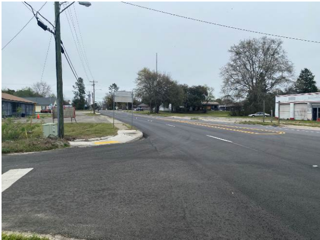
Main Hwy looking north
